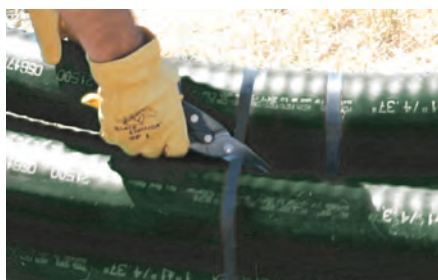
1 - Cut the three outermost fixing bands.
