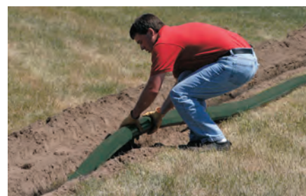
3 - Place ThermoPEX into trench.
